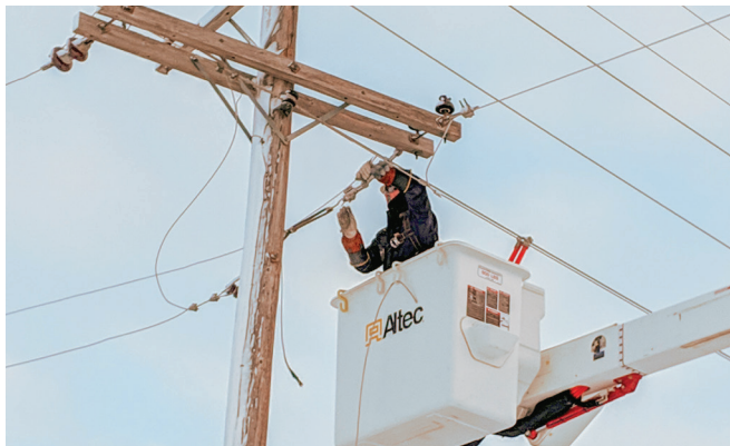
Journeyman Lineman Cody Ellis repairing lines after they were damaged during a storm this winter.
